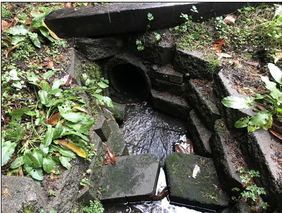
Photo 4. Stormwater channel flowing into 12" concrete stormwater main – private.
